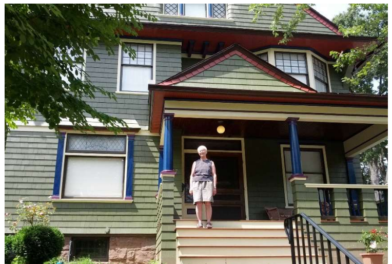
Summer of 2012, 67 Kenyon after renovations. Read about it on the website.
