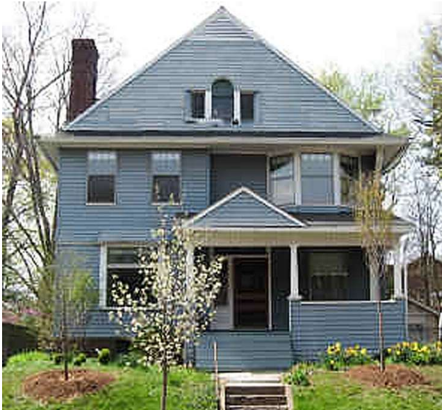
Aluminum siding of 67 Kenyon in 1975 hid all the detail
