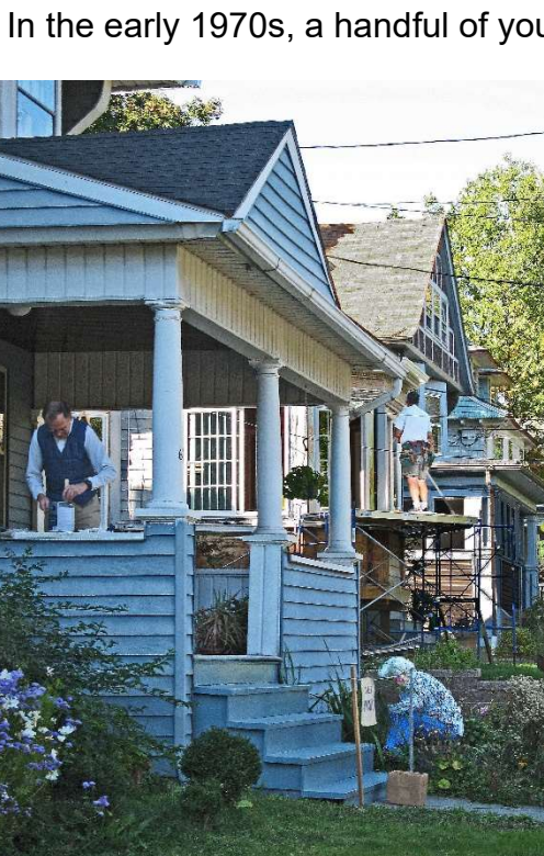
Figure 10- Working on homes
